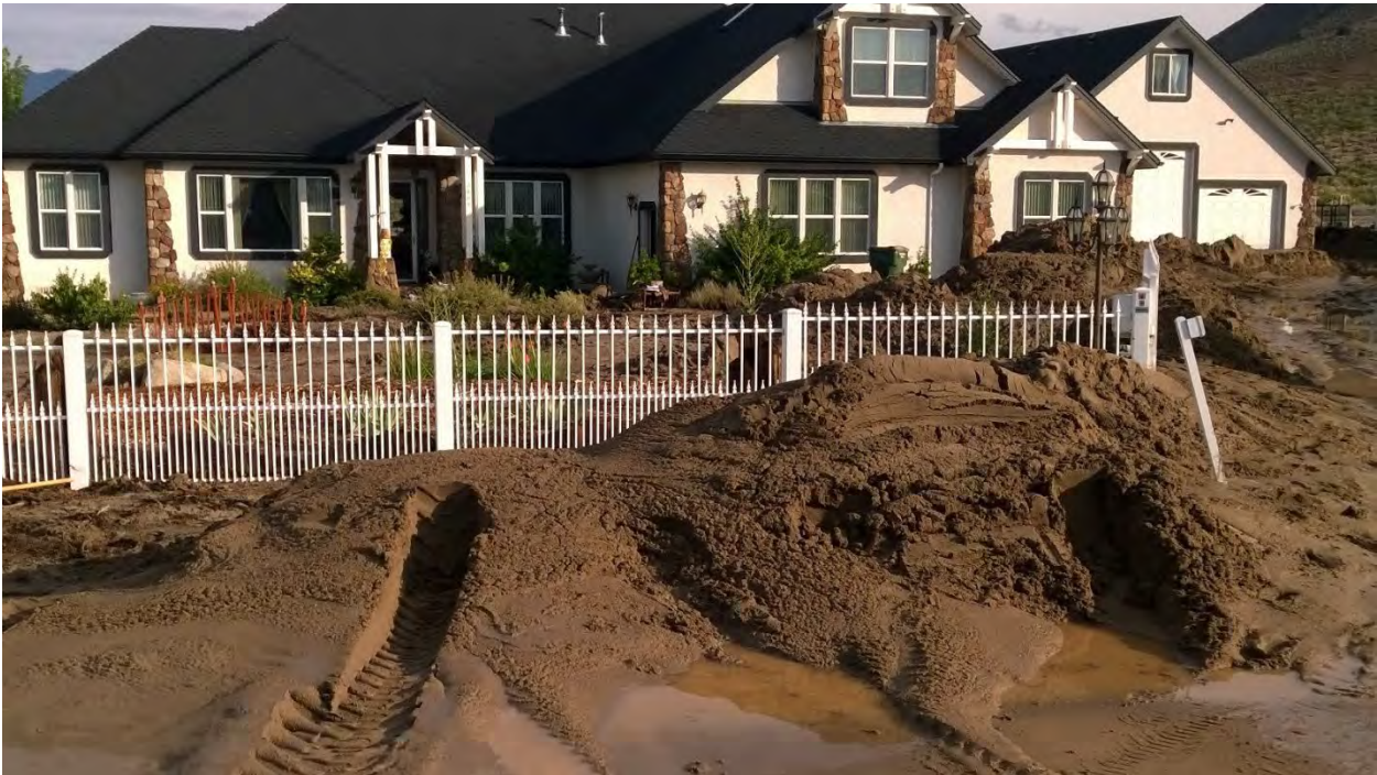
This property at the end of Mac Drive endured months of clean up after the July 2014 flood event.
